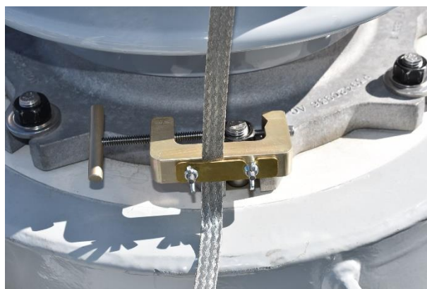
Earth connection to the ground clamp
